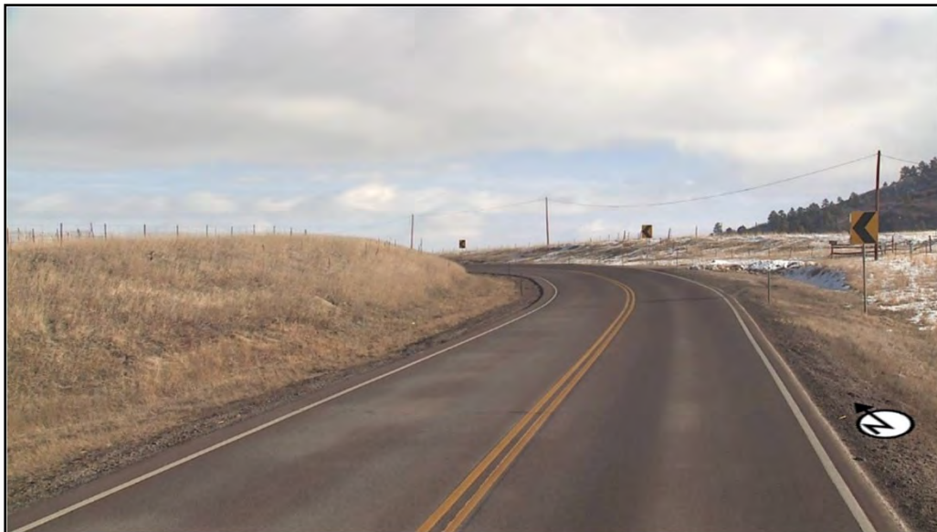
Figure A7: Northbound SH 83A at MP 32.25
